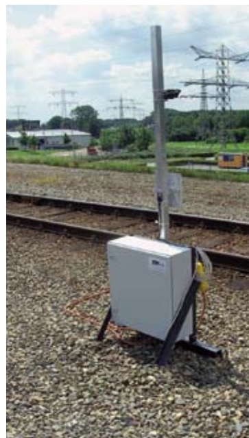
...and a reading device on the track at the Geleen plant
