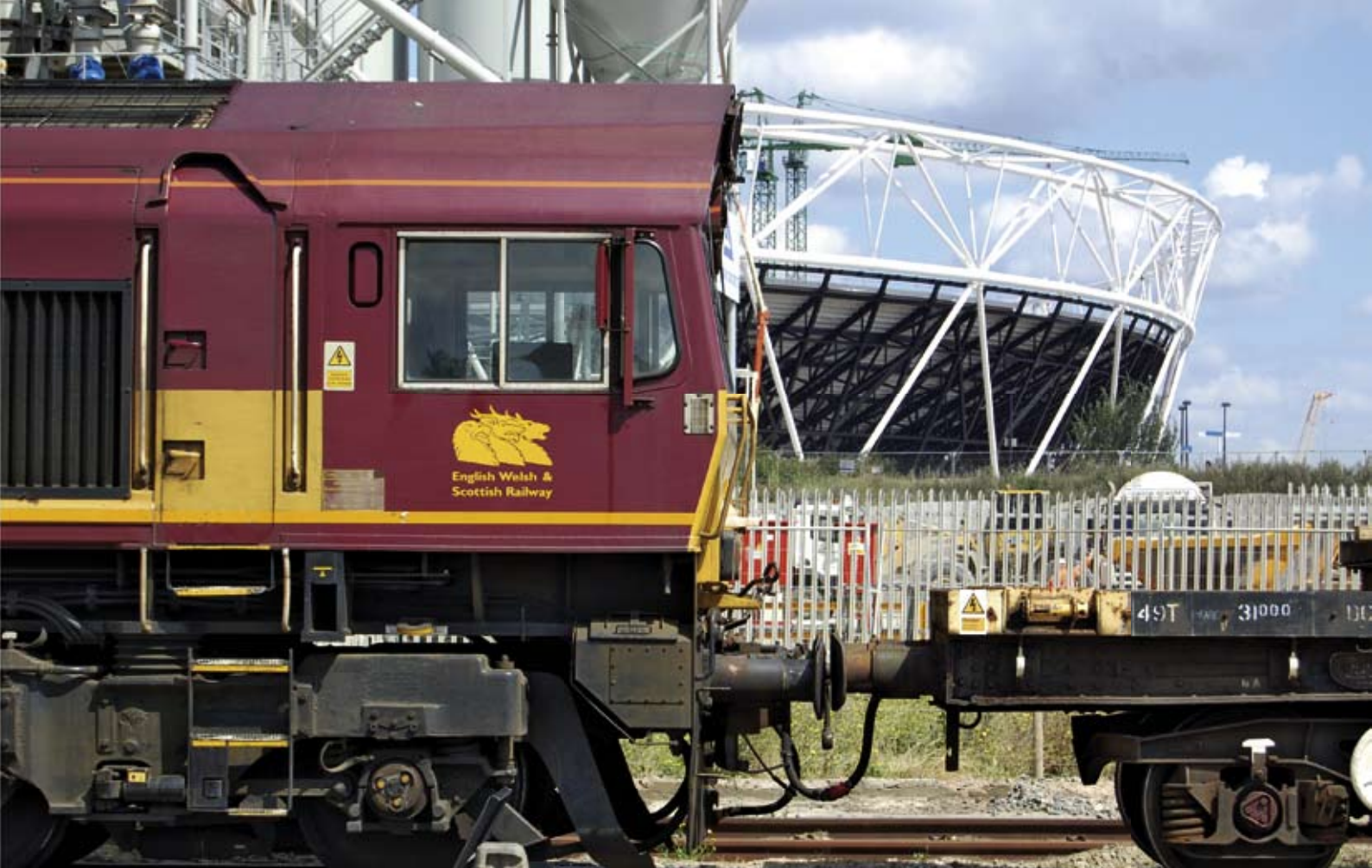
Huge construction site: the building materials reach the Olympic Park by rail
